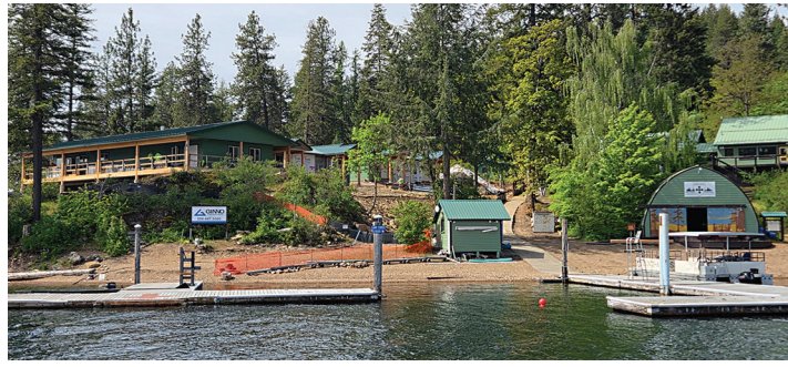
Camp Cross has building underway to expand cabins.
