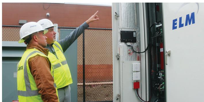
Avista workers inspect battery installed at MLK Center.
