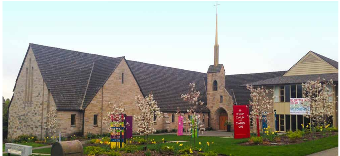
Magnolia UCC has redone its roof, insulation and lighting, qualifying for rebates. Photo courtesy of Magnolia UCC
