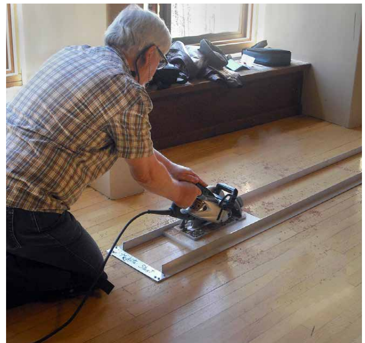
Dale Rominger and Charles Nishida cut grooves in floor for channels for wire. Below, Spencer Norby of Hearing Loop Northwest cuts grooves.
