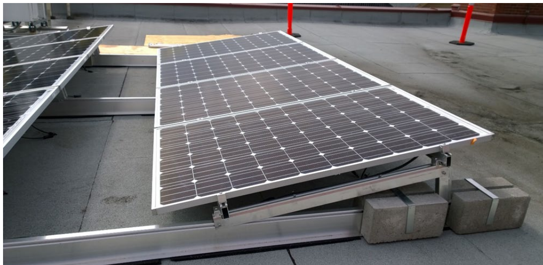
The solar arrays are 25.4 kilowatts, six times larger than most residences use.
